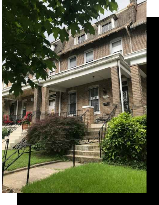
VIEW OF FRONT FACADE
